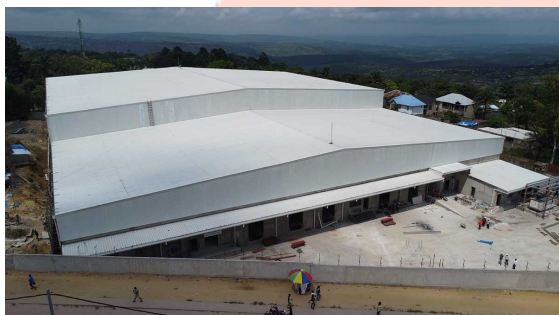
Prince Pharma Warehouse Kinshasa – DR Congo Fire Detection, Fire Fighting and Plumbing
