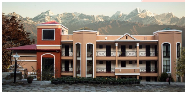
Bhangeri Darbar Resort – Nepal Fire Alarm System
