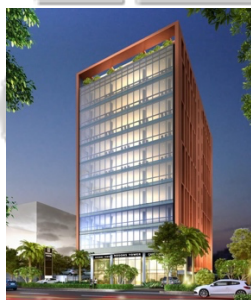
Roson Tower Kinshasa – DR Congo Fire Fighting and Plumbing
