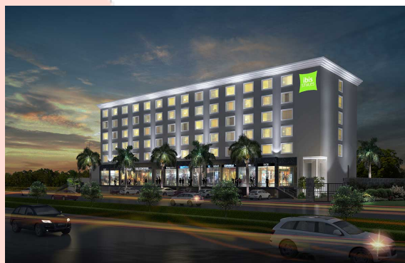
Regina Hotel Kinshasa – DR Congo Fire Fighting and Plumbing
