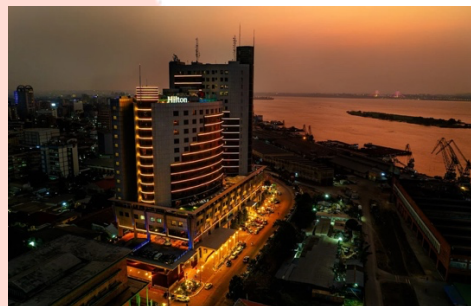
Hilton Hotel Kinshasa – DR Congo Fire Fighting and Plumbing
