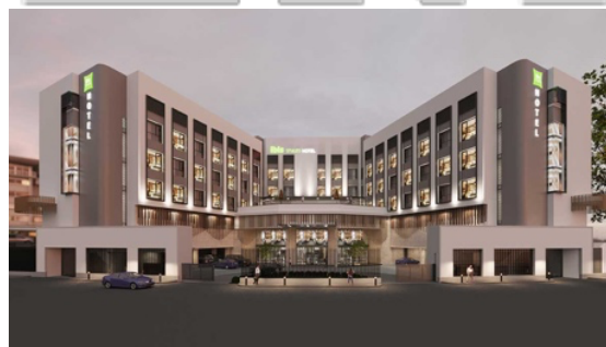
IBIS Hotel Goma – DR Congo Fire Fighting and Plumbing
